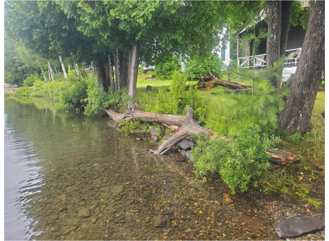
Lakeshore stabilization with pinned logs & native buffer planting.
