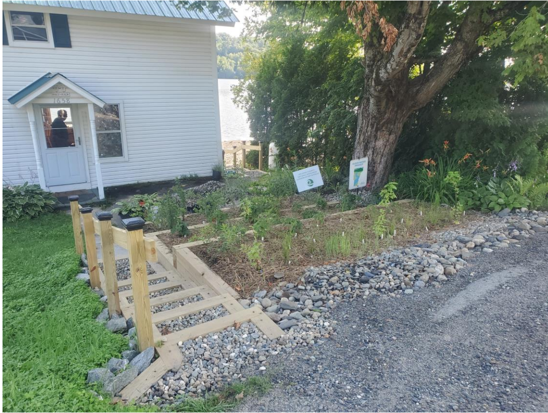
Infiltration steps & native bio infiltration garden bed install.
